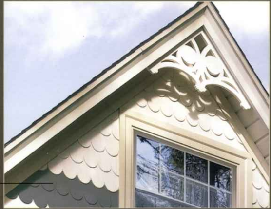
Combining Restoration Millwork architectural details in the scroll work and Vinyl Carpentry Half-Round Shingles creates a one-of-a-kind crafted look in the gable end.
